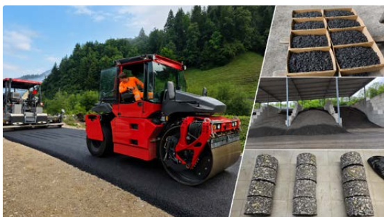
Field test section: paving, loose asphalt mix sampling and core extraction
