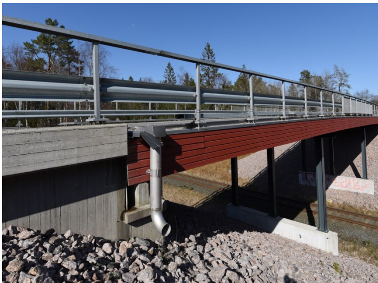
Figure 7. Good detailing of expansion joint drainage and down pipe.
