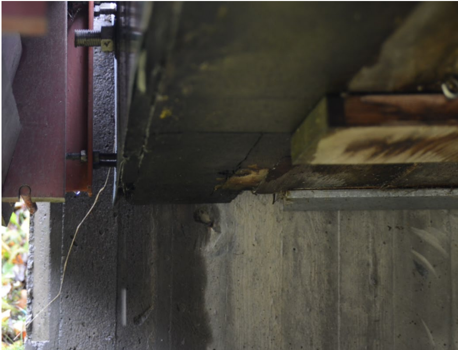
Figure 1. Wet outer beam from Klockarleden short.
