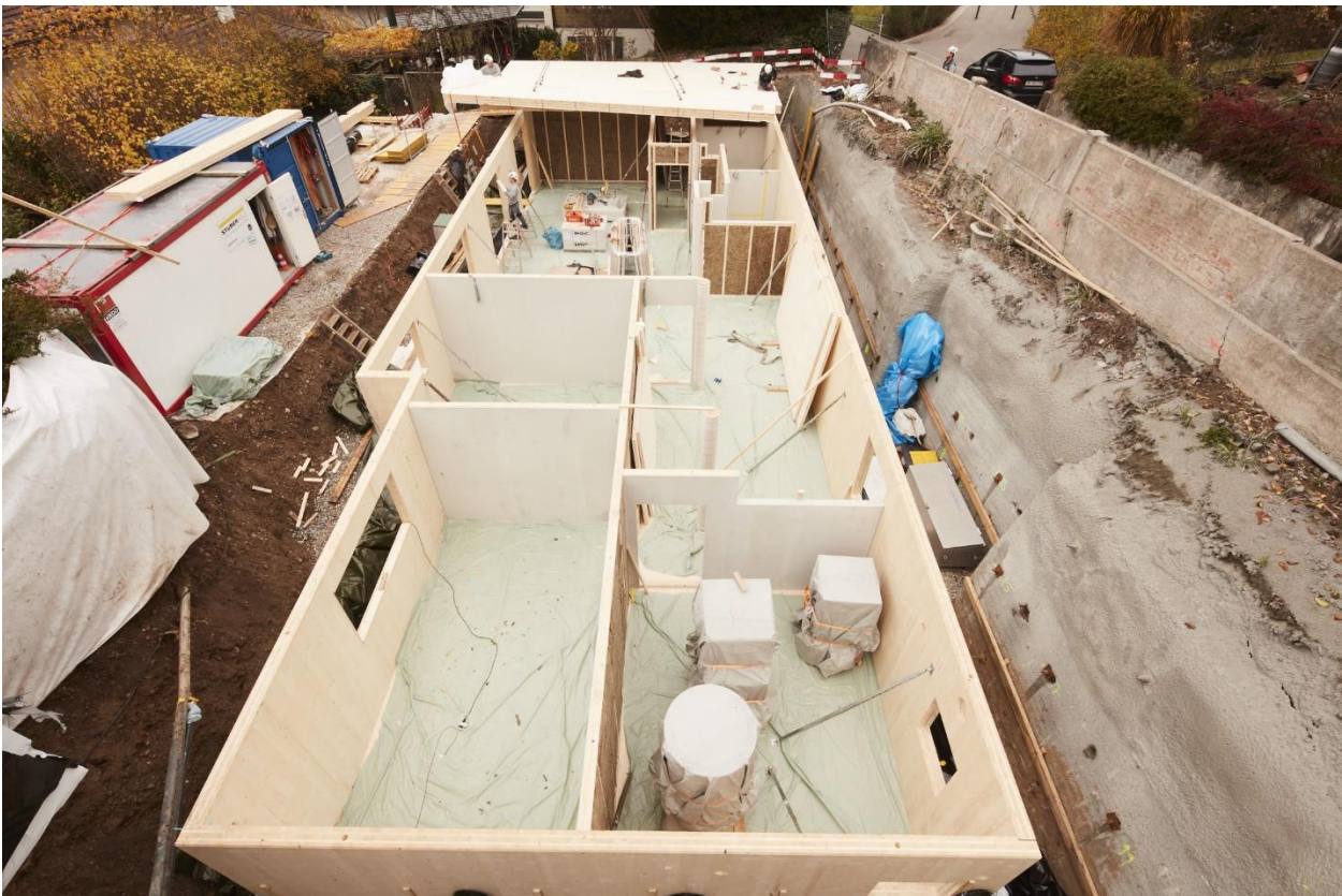
Timber basement, Source: www.timbatec.com
