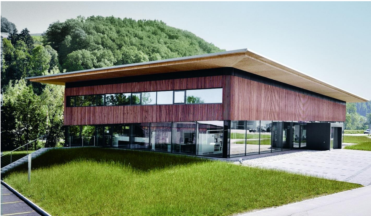
View of office timber building of Zaugg AG Rohrbach, photo Zaugg AG Rohrbach
