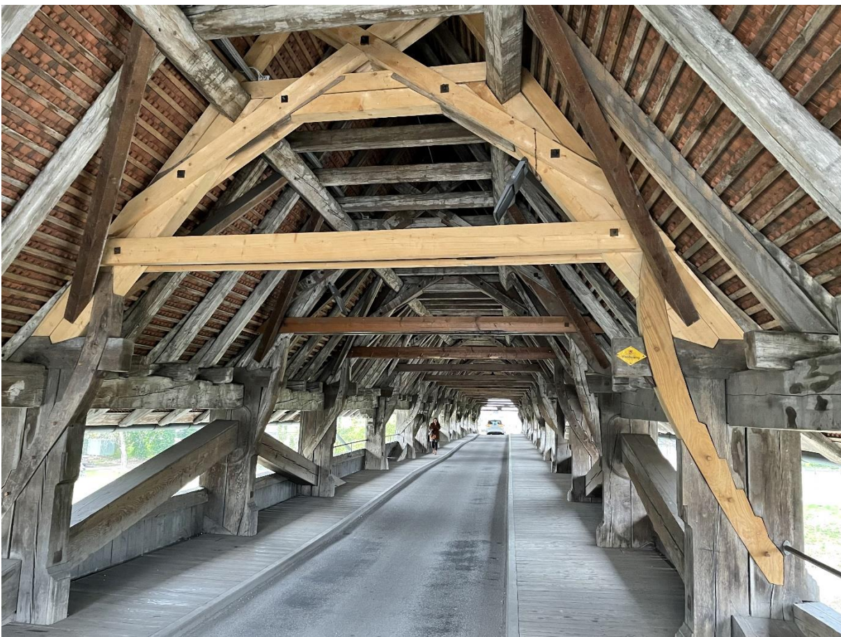
View inside of bridge Aarberg, photo S. Franke
