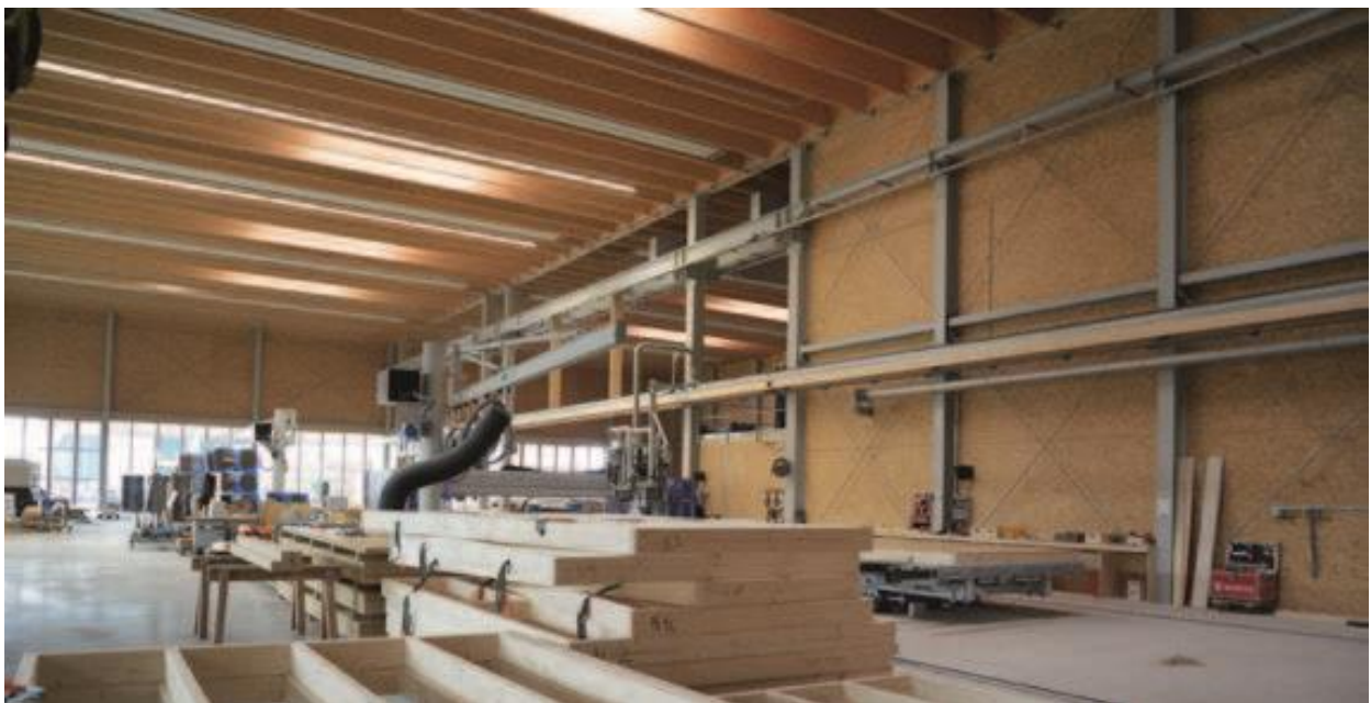
Inside view of the production hall, photo Zaugg AG Rohrbach
