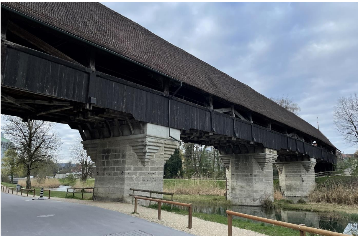
Side view with column heads of bridge Aarberg, photo S. Franke
