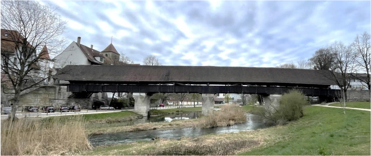
View of bridge Aarberg, photo S. Franke
