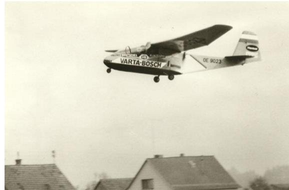
Figure 4: The HB ME-1 from Brdlitschla and Militky on his successful first flight on a man powered e-plane on 21st october 1973 in Wels (A)
