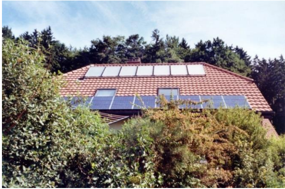
Fig. 6: Typical houses of a solar energy consumer around the year 2005. The hot water solar thermal device (left picture) cost about 15'000 sFr. (or US$). The 6 kWp PV plant (right picture) was about 50-60'000sFr. (Photos: Muntwyler).
