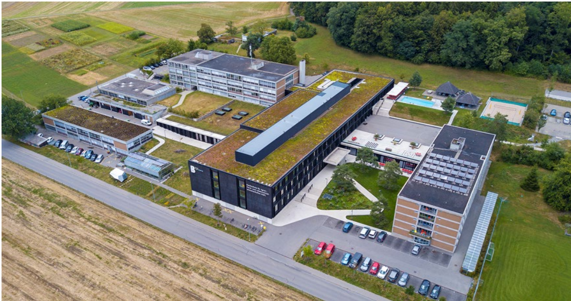
Picture: Campus HAFL
