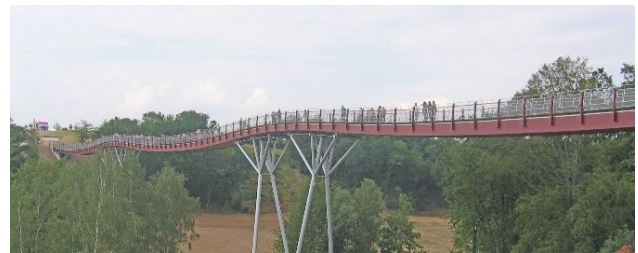
Figure 2: Stress-Ribbon-bridge Gera-Ronneburg (GER)
