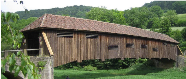
Figure 8: Bridge Unterregenbach (DE)
